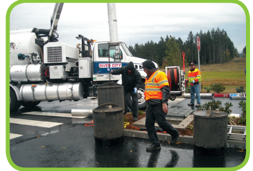
BayFilter System Cleanout
