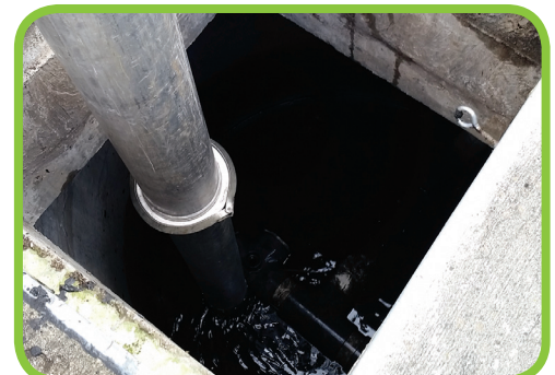
Jet Vactoring Through Access Hatch
